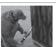
**Step 10 - Caulking:** Caulk the top of the door drip, all the corner moldings, roof corner seams and wall seams.
